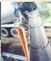
Pouring SCLC into Insulated Concrete Forms From a Concrete Truck
