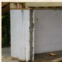
Exposed Hardened SCLC at the Wall End
